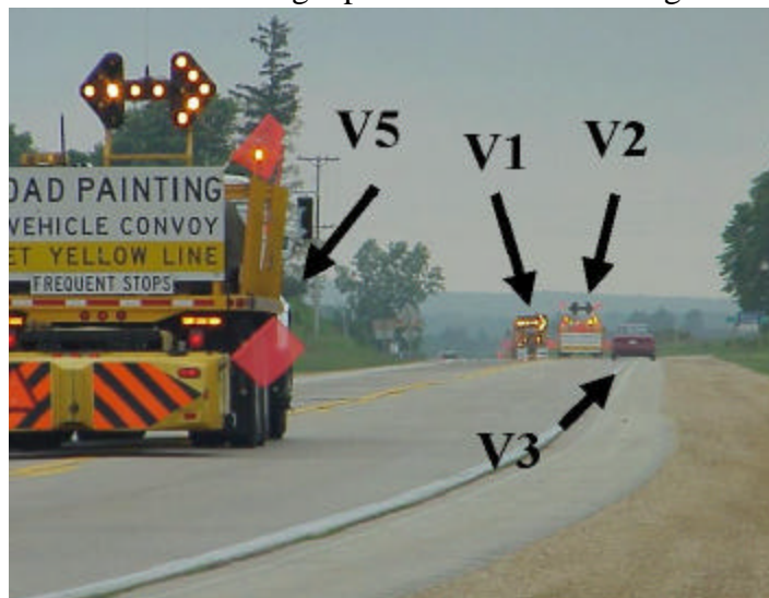
Figure 8. View of Painting Operation Vehicle Arrangement
