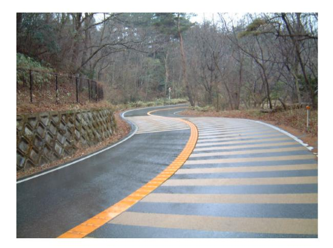
Typical anti-skid pavement install section.
