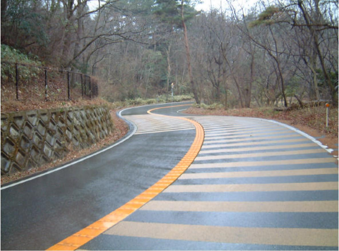
Typical anti-skid pavement install section.
