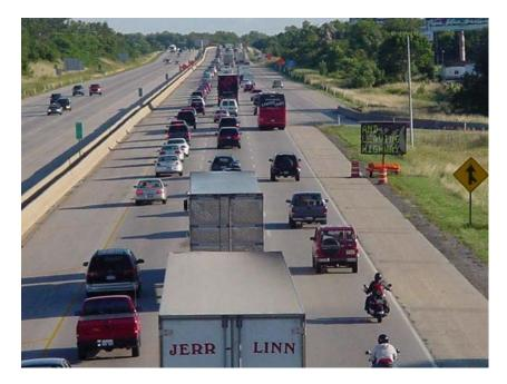
Picture C2. I-94 Southbound Racine County. Construction Phase One: Left Half of Travel Lanes Removed, Right Shoulder Rumble Strips Patched Over with Asphalt
